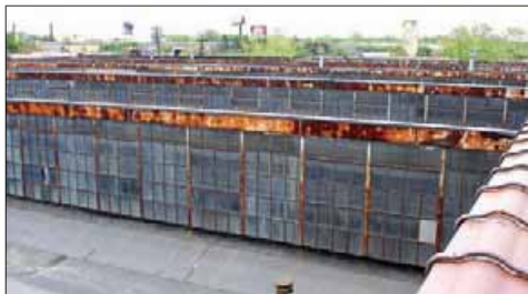
The aged saw-toothed roof in a current photo. Designed to provide maximum natural heat and light, the exposed windows proved to be a maintenance nightmare. Buckets were often required on the factory floor to catch rainwater from the leaking windows.
